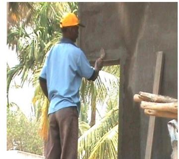
On smooth concrete walls, the rendering coat shall be dashed on to ensure adequate bond. The dashing of the rendering coat shall be done using a strong whipping motion at right angles to the face of the wall, or it may be applied with a plaster-machine or cement-gun. In either case, the plaster shall be projected on to the surface with considerable force.
