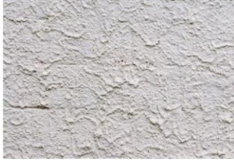
**Rough cast finish:** Mortar used to get rough cast finish consists of coarse aggregate (CA)/gravel along with cement and sand. Their ratio cement : sand : coarse aggregate is about 1: 1.5: 3. The size of coarse aggregate used is 3mm to 12mm. Large quantity of mortar is taken by trowel and it is dashed into the surface and levelled using wooden float. Usually this type of plaster finish is preferred for external renderings. This finish is durable as well as decorative.
