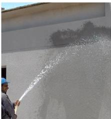
Curing shall be started immediately after stiffening / hardening of the plaster surface. The plaster shall be kept wet for a minimum of 10 days during which period it shall be suitably protected from any damages. Curing is generally carried out by regular spraying of water without allowing the surface to dry at any point of time. Improper or irregular curing may lead to crack formation in plaster work.
