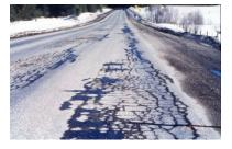
Air entrainment can be improved by optimizing the mixing time and reducing the concrete temperatures. Type of cement and cement content also influences the volume of air entrainment. Air entraining admixtures can prevent this type of deterioration by incorporating millions of tiny, discrete air bubbles in the concrete.
