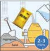
Mix cement, sand and aggregates, as per the mix design.
