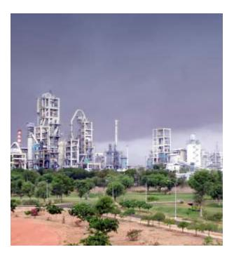
Based on the evaluation, in-house modification, conversion of ESP to bag house and utilisation of latest technology like high frequency convertor, were planned for reducing the dust emission level. The decision to upgrade the equipment was taken on a case-to-case basis. The reduction of emission level was targeted to less than 30 mg/Nm3 for each plant from the present level.
