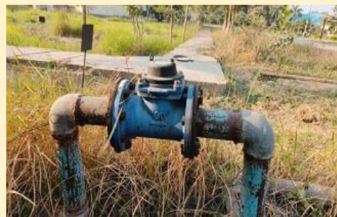
SAMPLE WATER FLOW METER INSTALLED AT BOREWELL
