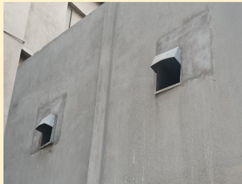
Ventilation fans installed at various places in plant
