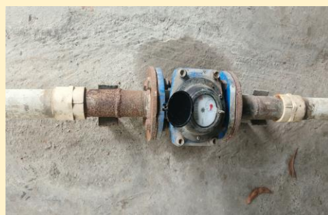
SAMPLE WATER FLOW METER INSTALLED AT BOREWELL
