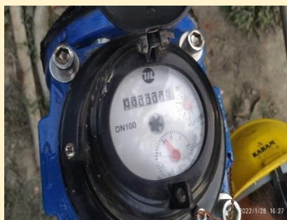
SAMPLE WATER FLOW METER INSTALLED AT BOREWELL
