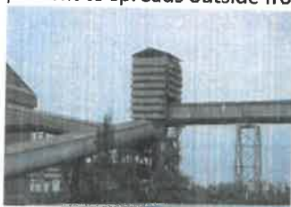
Covered belt conveyor and Bag Filter
