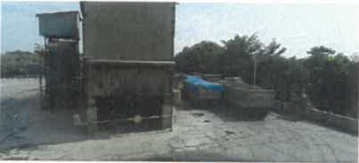
Mechanized truck tippler equipped with bag filter and curtain
