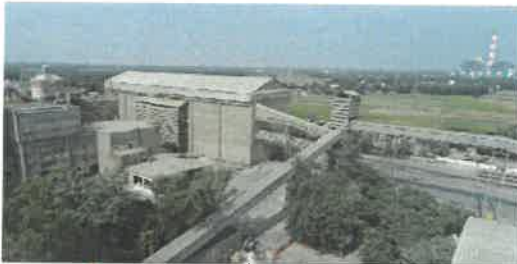
Covered storage shed and conveyor belts
