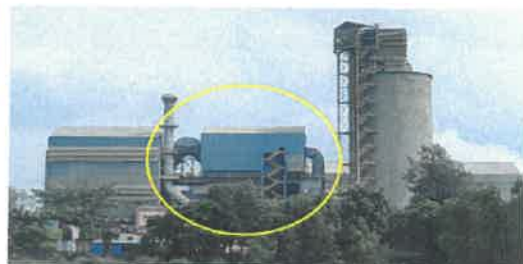
Bag House attached with cement mill stack
