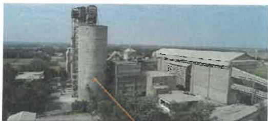
Cement storage silo
