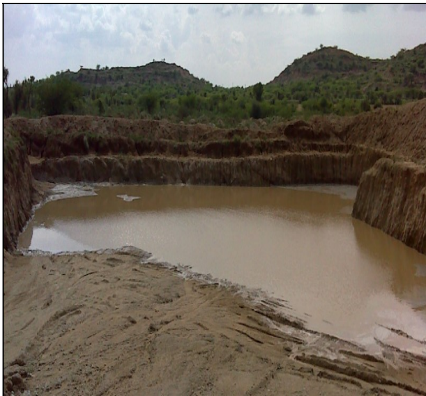
Recharge Pit developed in Mines
