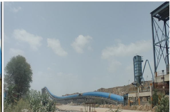
Covered conveyor belt from crusher to Plant
