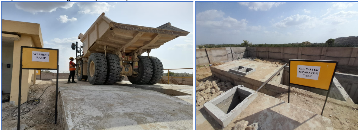
Mines Workshop Vehicle Washing and Oil & Grease Trap
