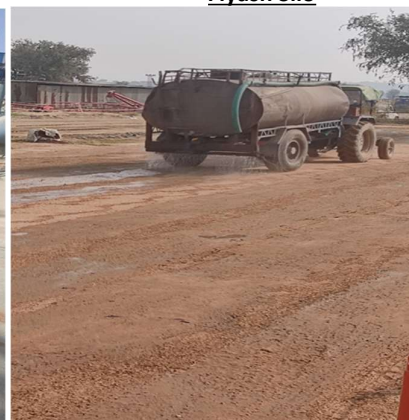
Water Sprinkling arrangement
