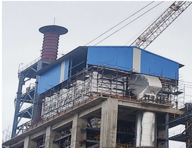
Coal Mill – Bag House with Stack
