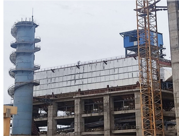
Cement Mill – Bag House with Stack
