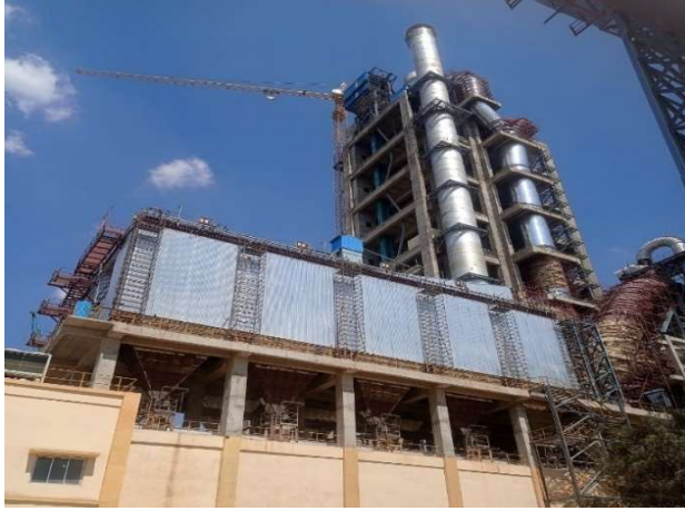
Kiln & Raw Mill – Bag House with Stack
