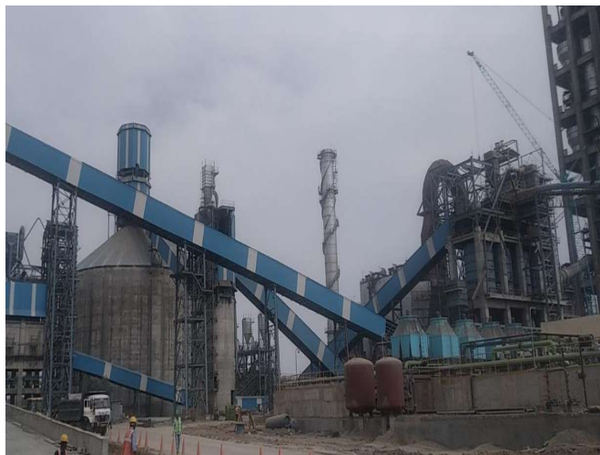
Covered Conveyor Belts for material transportation
