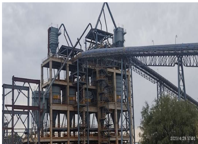
Bag Filters at Material storage & transfer points
