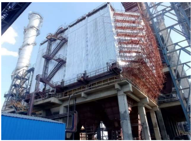
Clinker Cooler- ESP with Stack
