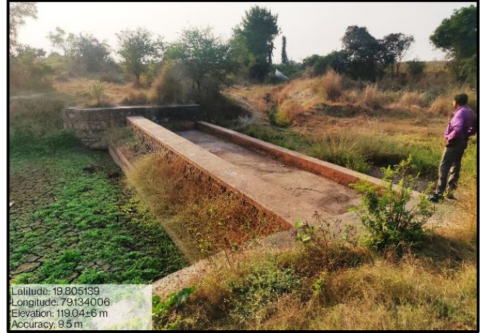
Check dam, Village: Awalpur
