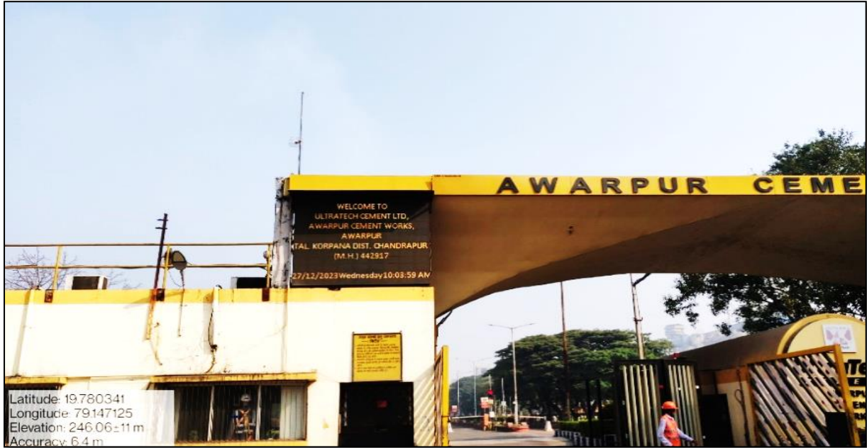
Digital Display Board installed at main gate
