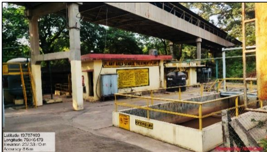
Sewage Treatment Plant at Plant
