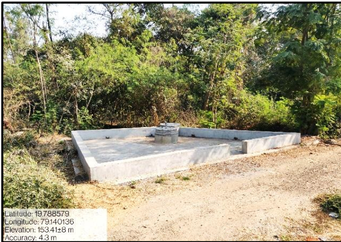
Behind Unit Head Bungalow
