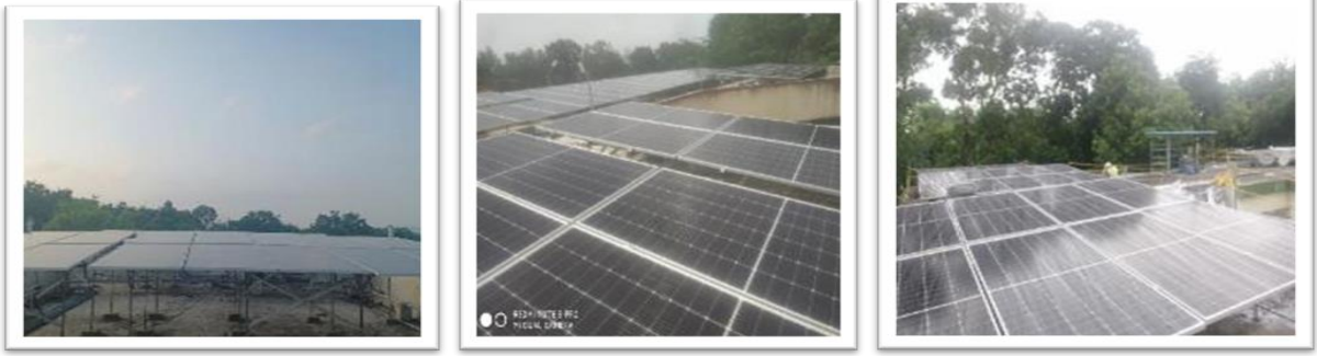
482 KWp Roof top Solar plats power Generating Power 1.5 to 2.35 MW/day
