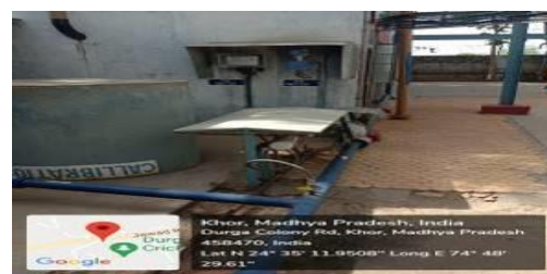
Online PH & Turbidity meter fitted at STP
