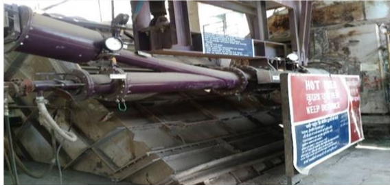
Installation of Low NOx Burner
