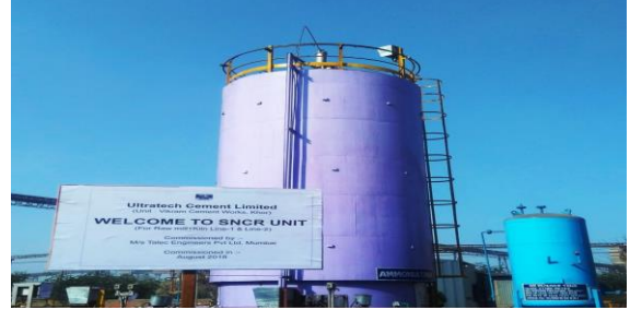
Installed Selective Non catalytic Reduction (SNCR)
