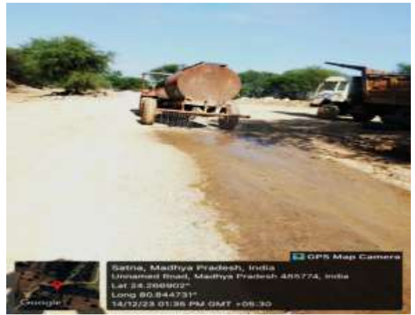
Water spraying at the time of limestone loading
