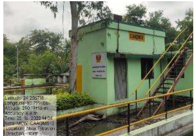
CAAQMS-2, At Filtration Plant
