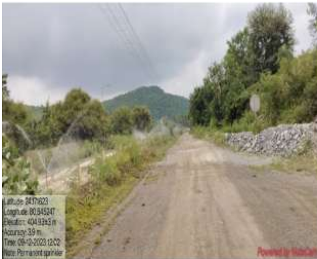
Permanent Water Sprinkler at haul Road
