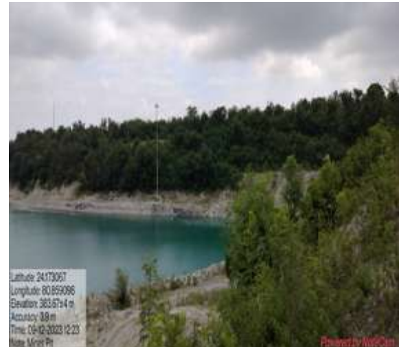
Water reservoir in ML Area
