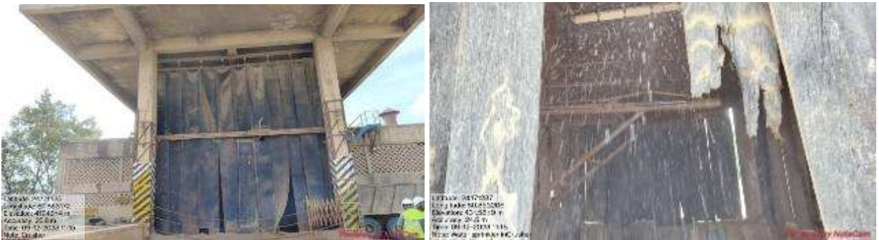
Fully Covered Crusher with mist water spray system
