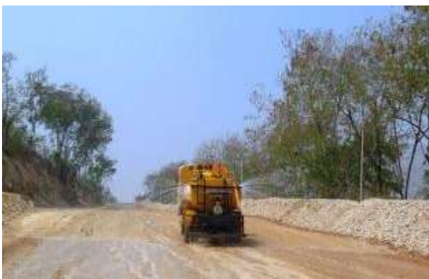
Water tanker for spraying on haul roads
