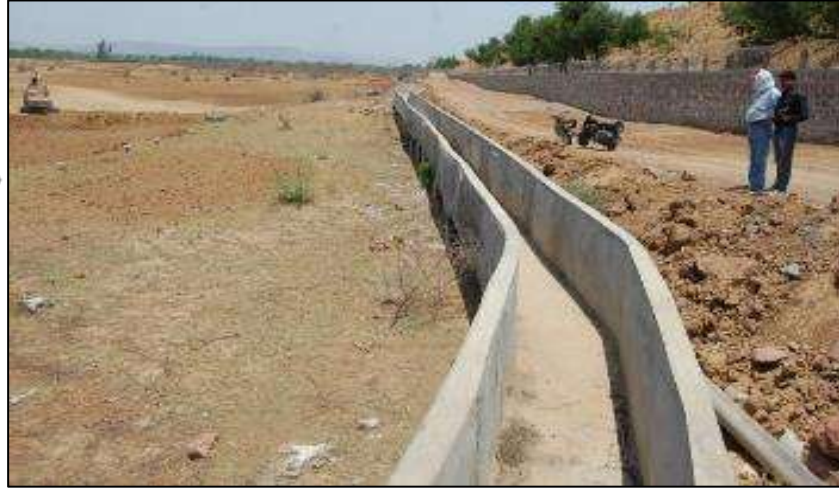
Rain water Collecting channel to Reservoir & Recharge Shaft
