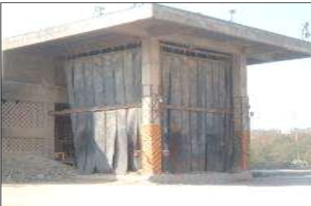
Rubber curtains at Dump hopper and atomozed water spray
