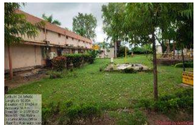
Roof top water harvesting
