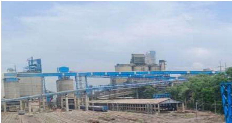
Cement/Clinker Bulk loading Silo
