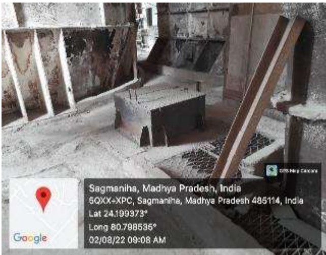
AF feeding Hopper at Line-3
