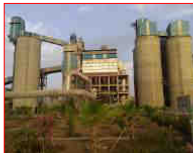
Fly ash & Cement Storage Silo's
