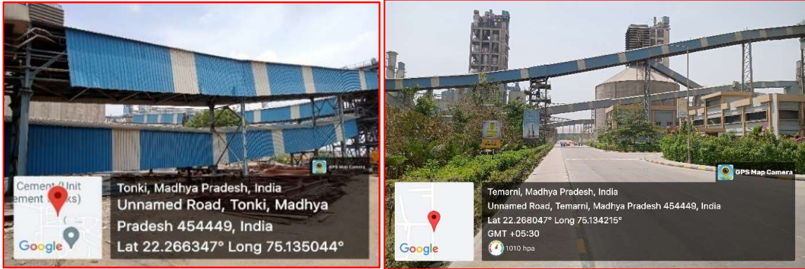
All the material transportation belts are fully covered
