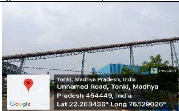
Material transfer through Belt.
