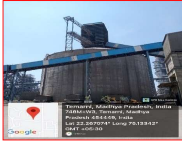
Silo for Storage of Clinker L-1
