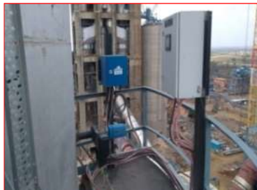
Opacity Meter (PM) L-1 Cooler ESP Stack
