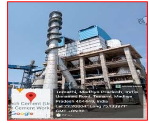
Cement Mill-3 Baghouse
