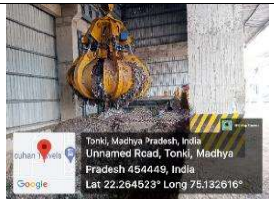
Grabber feed Material at hopper
