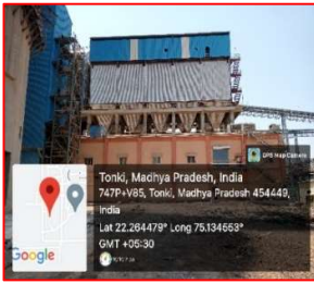
Line-2 Raw Mill Baghouse
