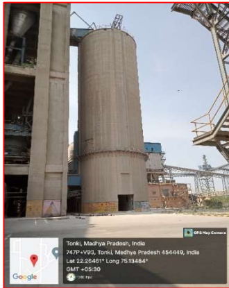
Line-2 Raw Mill Storage silo
