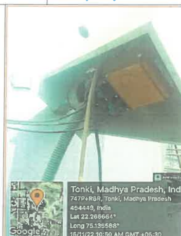
Line-2 Cooler ESP Stack Opacity Meter
