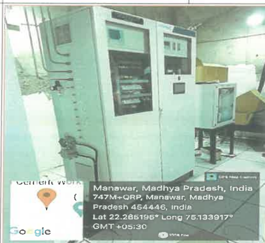
Line-2 Raw Mill & Kiln Bag house Stack Sox , NOx and PM Analyser
