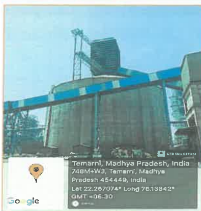
Silo for Storage of Clinker L-1
