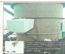
Line-2 Coal Mill Baghouse Stack Opacity Meter
