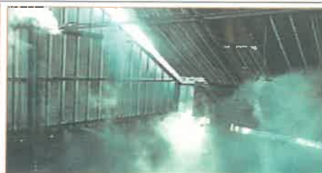
Water Sprinkler for Coal Unloading
