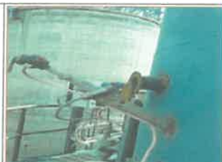
Cement Mill - 2 Bag house Stack Opacity Meter
