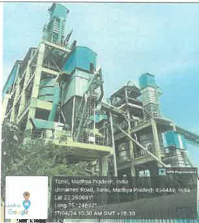
Bag Filter provide at transfer point
