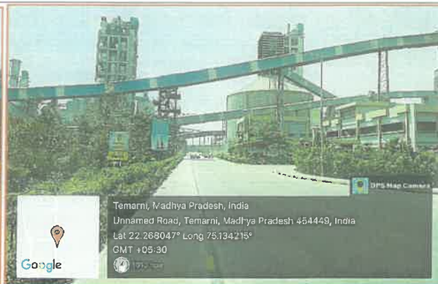
All the material transportation belts are fully covered
