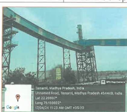
Covered conveyor belt with bag filter
