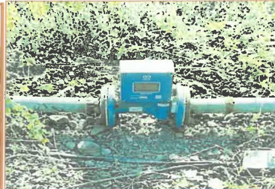
Photographs of Digital Flow Meters
