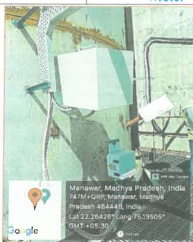
Line-2 Raw Mill & Kiln Bag house Stack Sox , NOx and PM Analyser
