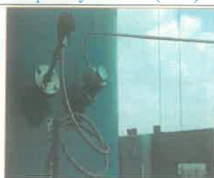
Line-1 Coal Mill Bag house Stack Opacity Meter
