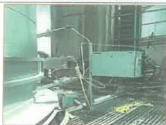
Line-1 Raw Mill & Kiln Bag house Stack Sox , NOx and PM Analyser
