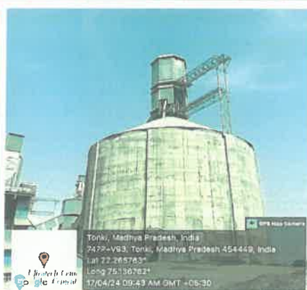
Silo for Storage of Clinker L-2
