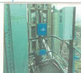
Line-1 Cooler ESP Stack Opacity Meter
