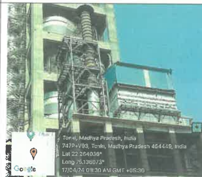
Line-2 Coal Mill With Baghouse
