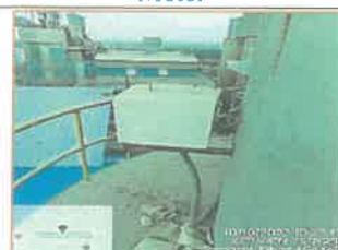
Cement Mill-3 Bag house Stack Opacity Meter
