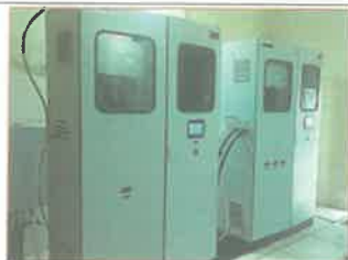
Line-1 Raw Mill & Kiln Bag house Stack Sox , NOx and PM Analyser
