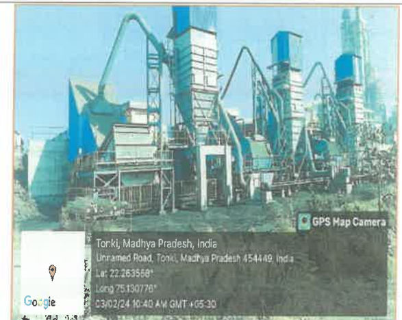
Installed bag filter at transfer point
