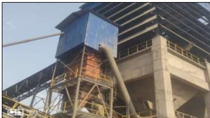
Installed Bag Filters
