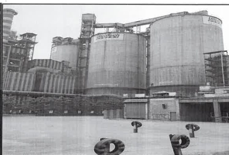
Closed Silo for storage of Cement/Clinker/Fly ash
