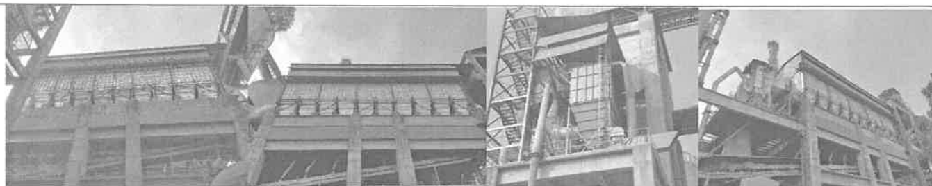
INSTALLED AIR POLLUTION CONTROL DEVICES – BAG HOUSE
