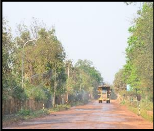
Water Sprinklers installed on Haul Road
