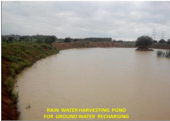
Rehabilitated old mined out pit converted into a water reservoir
