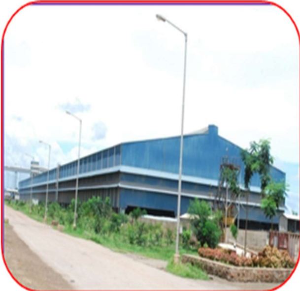
Closed LS Shed-Phase II
