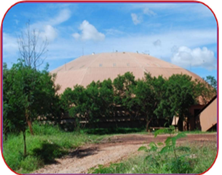
Closed LS Shed - Phase I
