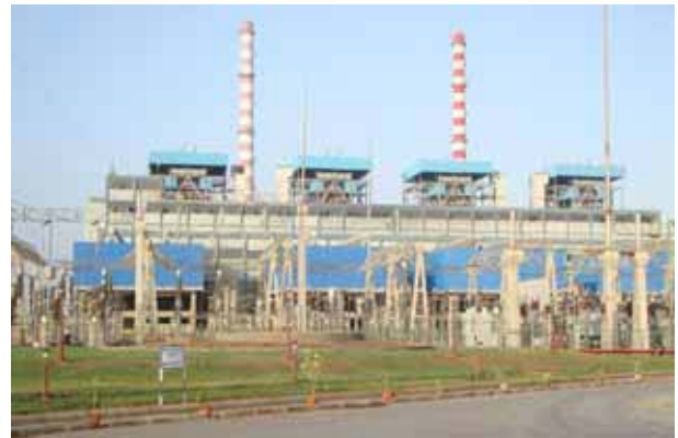
Captive thermal power plant at GCW
