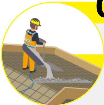
If the slab is sloping, always start the work from the side of a slope.
