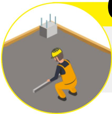
Firstly, get the screeding done. In screeding, the upper layer of the excess concrete is removed. This gives us levelled surface.
