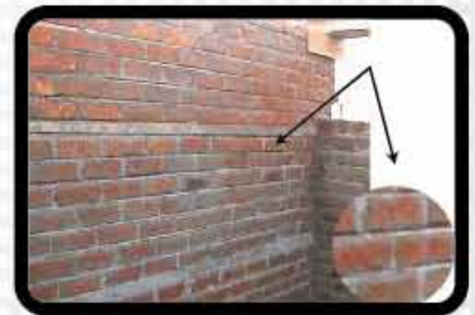
Raked Brick Masonry
