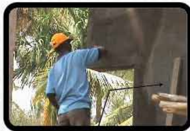
Finishing using WOODEN FLOAT
