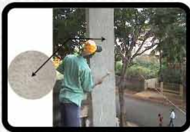
Hacking of Concrete surfaces
