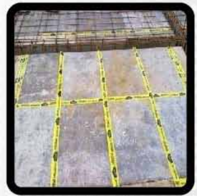
Joint Sealed With Mastic Tape
