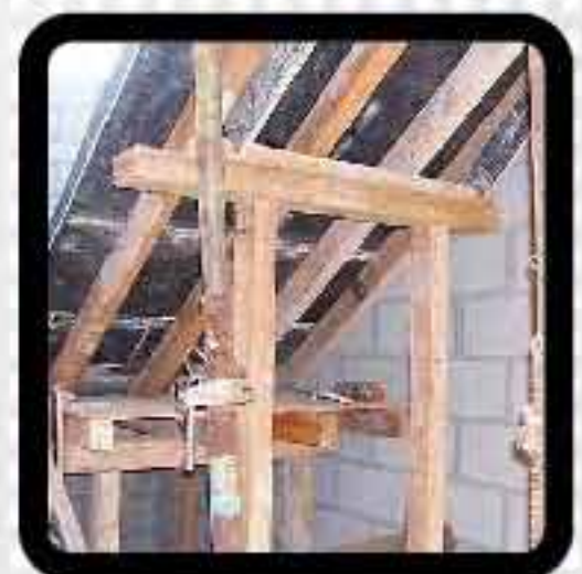
Well Supported Stair Formwork
