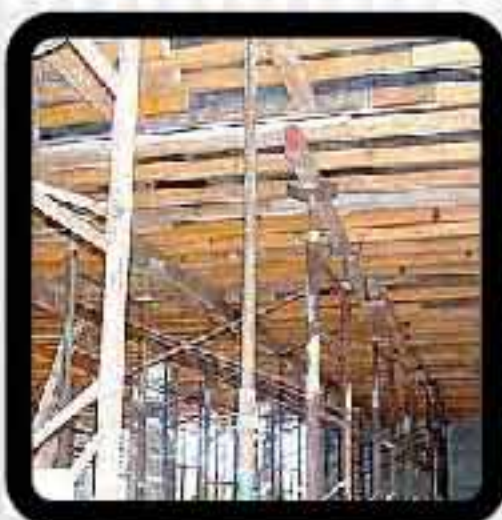
Well Braced Formwork with Steel Props
