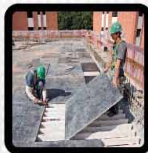
Slab Formwork
