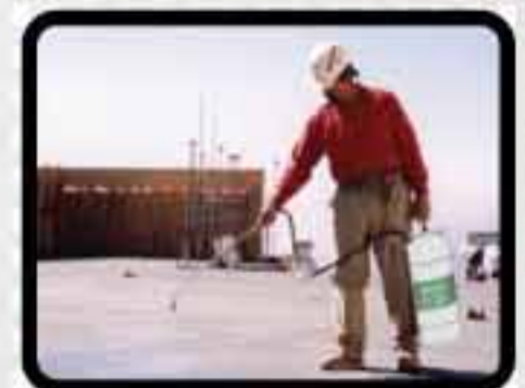
SPRAYING/SPRINKLING For Plastering & Masonry
