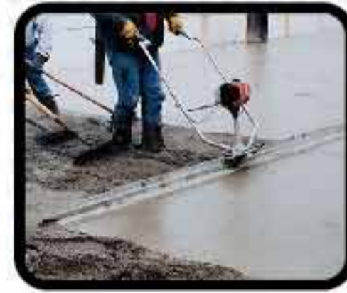
Compaction - Using Screed Vibrator
