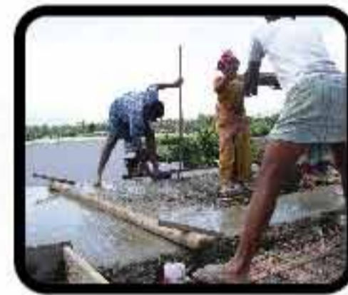
Tamping - Using Wooden Cross Beams of Size 10x10 cm
