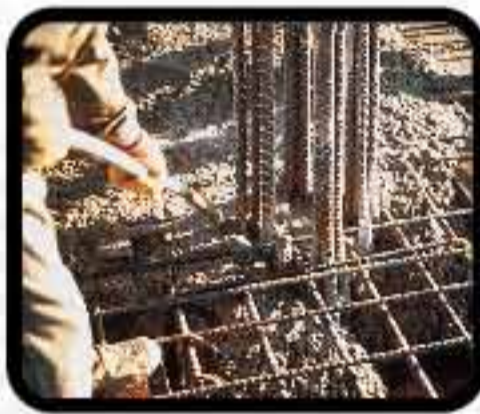
Rodding - Using 2m Long, Iron Rods/Wooden Ballies
