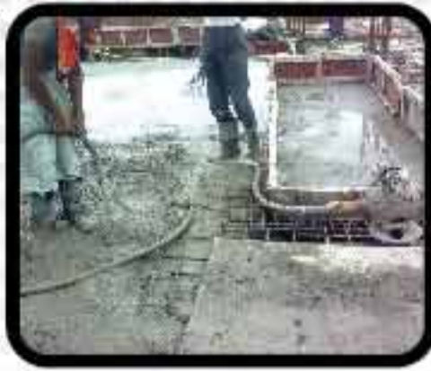
Compaction - Using Needle Vibrator of dia 20mm
