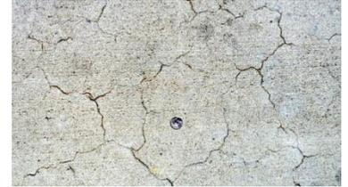
Generally craze cracks develop at an early age and are apparent the day after placement. The crazing is more prominently seen when the surface is wet.
